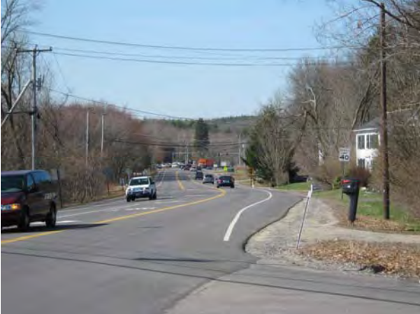
NH Route 111 Looking West from No. Lowell Road
