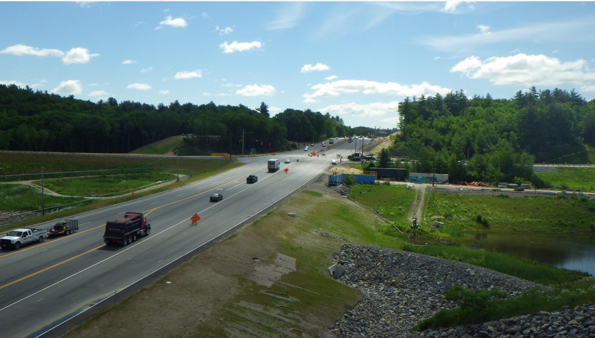
NH Route 111 Facing East, Exit 3 Area at the NB Ramps Intersection
