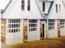
The vinyl panels over the steel doors have a wood grain.
